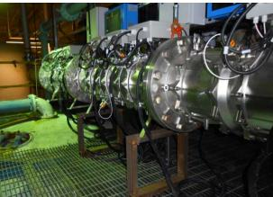
Incorporating HOD™ UV at Plant Bowen has reduced the use of SMBS for dechlorination and minimized the frequency of micron filter replacement.
